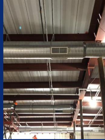
Spiral duct installed in gymnasium
