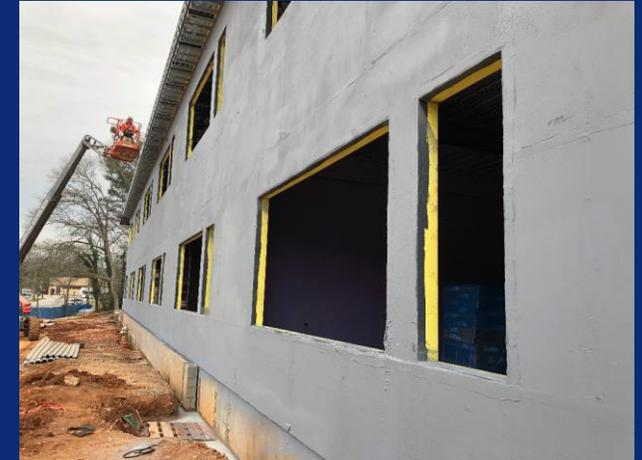
East side north elevation waterproofing applied
