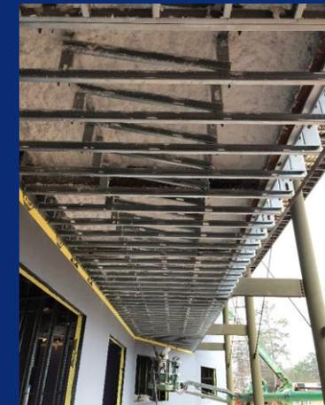
Spray in insulation ongoing in soffit outside of reception
