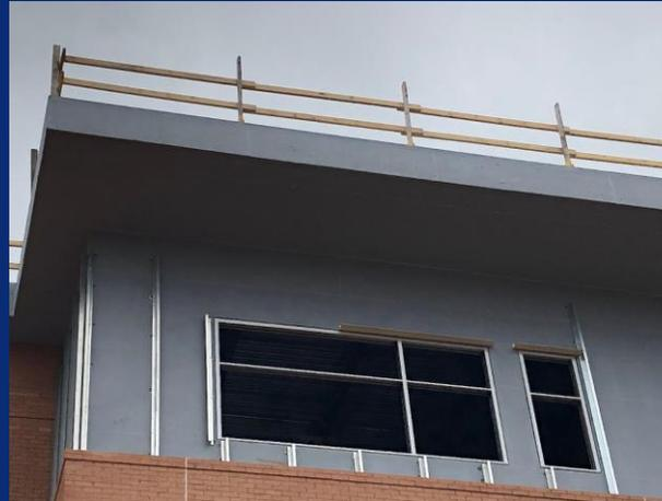
Metal panel install beginning on southern exterior of 3<sup>rd</sup> level
