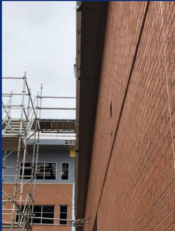
Soffit panels installed on perimeter of gymnasium and cafeteria
